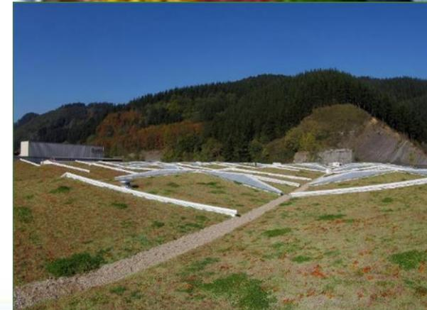
Green Roof on this lightweight production facility in Spain helps reducing solar radiation transfer into the building. Up to 40% energy saving for air-conditioning can be reached during the summer periods.
